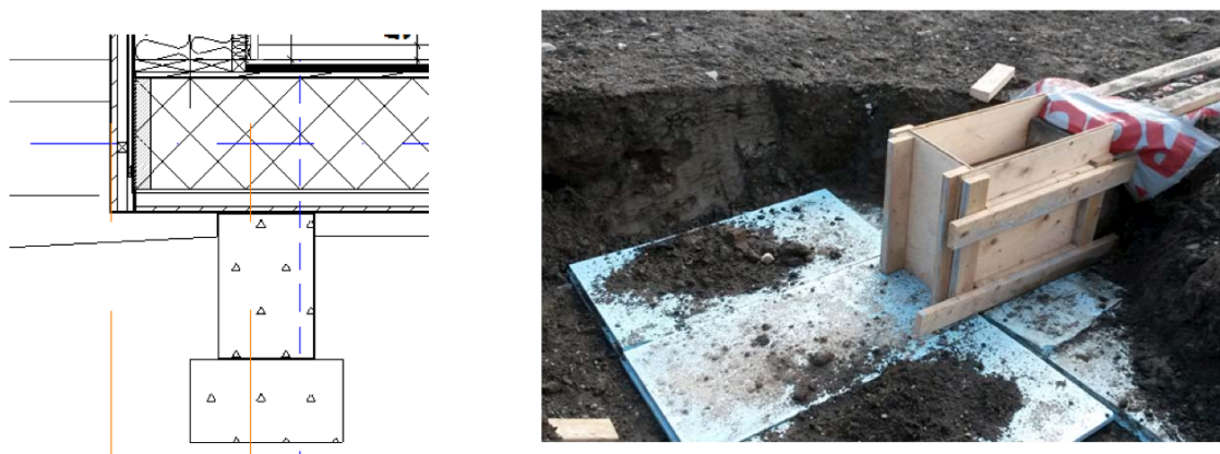
The sketch is from the design stage (courtesy of Bergersen Arkitekter AS), and the photograph (courtesy of Marianne Rose Inman) is from the construction/as-built stage. Note the missing concrete pier foundation and additional insulation.
